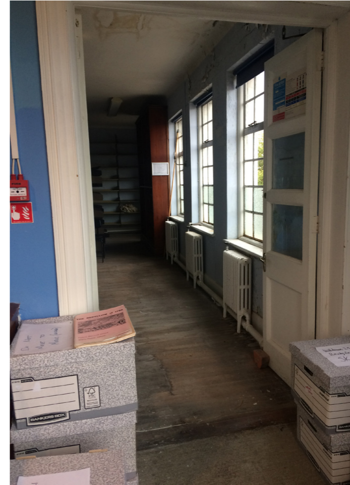
Existing radiators and associated pipework to be removed
