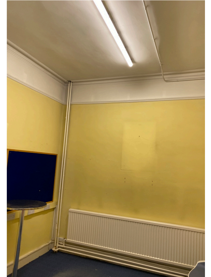
Existing radiators to be removed
