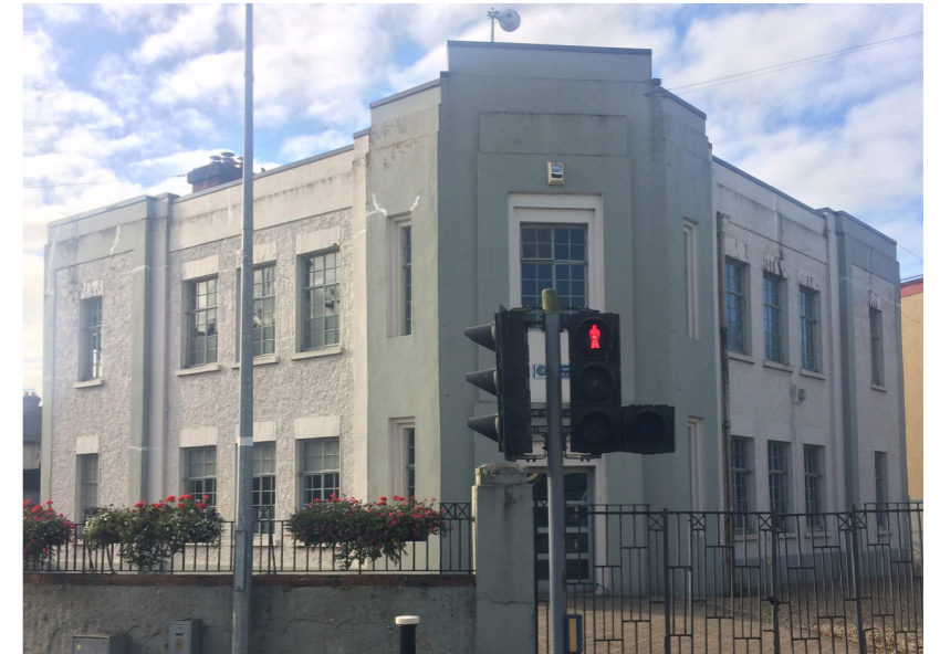
1. Profiled parapet walls
