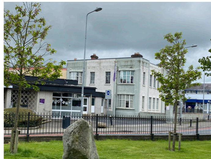
Above; Three of the 4 uPVC window units to be replaced can be seen, The fourth is obscured by the 1970's building
