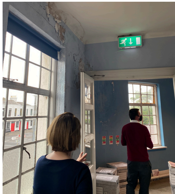
Door at 1F level between Teaching learning room and stair
