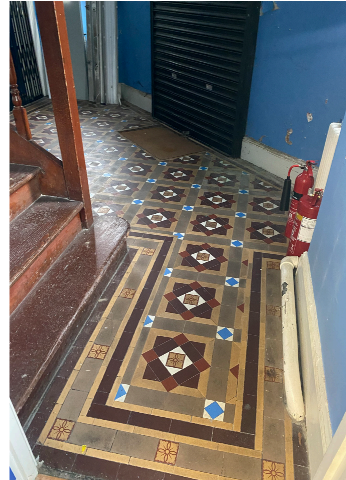
Existing heating system pipework to be removed
