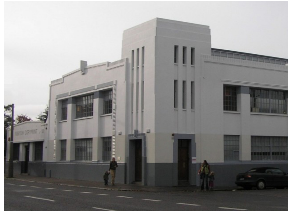
The Kodak Building - strong corner and stepped parapet
